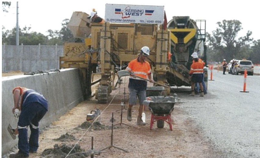
Figure 6: Typical machinery for slipform barrier construction
