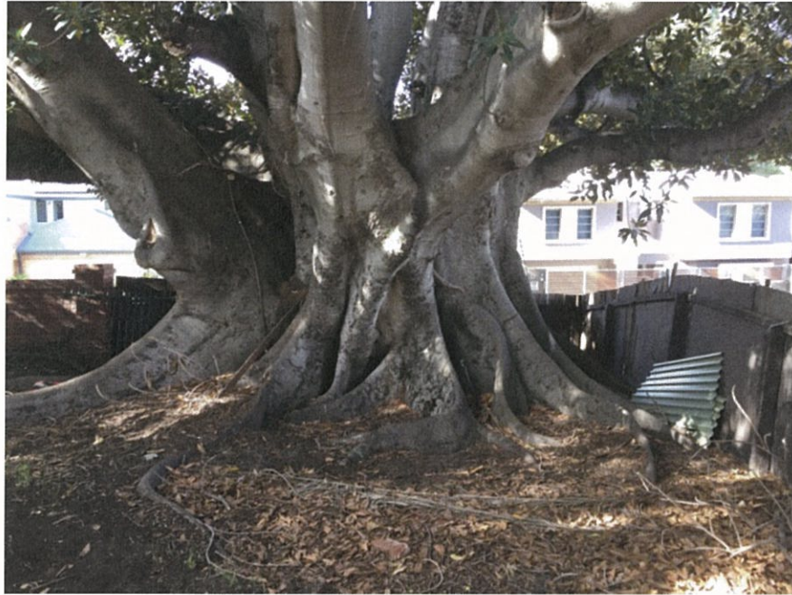
Figure 3. Sounding with a nylon hammer at the trunk basal area failed to return any tonal variations indicative of a thin residual trunk wall or internal wood decay and no significant radial cracking or cavity openings were evident; looking towards the east.
